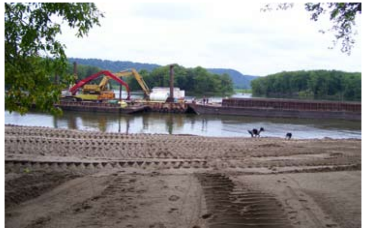
Sand added to Wisconsin Beach at Mile Marker 664.6 makes the beach area more stable and useable for beach goers.
